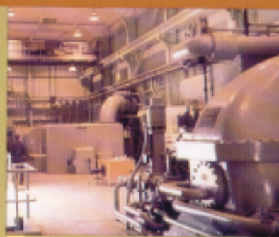
Circa 1960's – Two 27.5 MW turbine-generators with 22-inch last stage blades in a northern California utility geothermal power plant.
